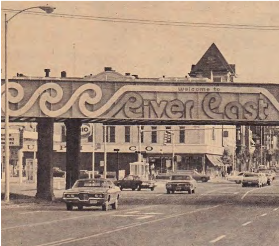
Rail viaduct over Main Street, image from 1978
