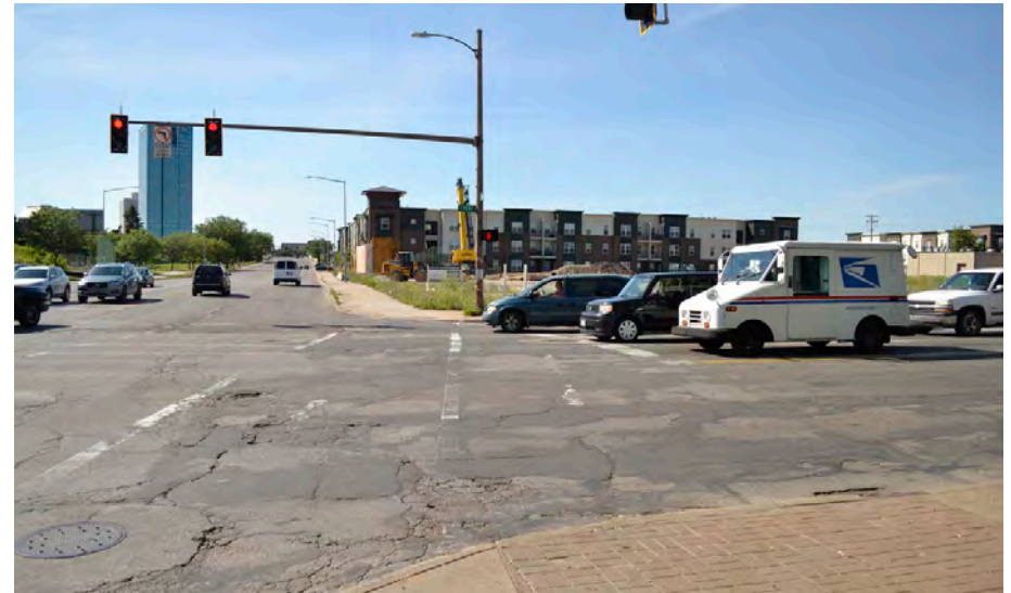
Intersection of Main and Front Street looking west .
