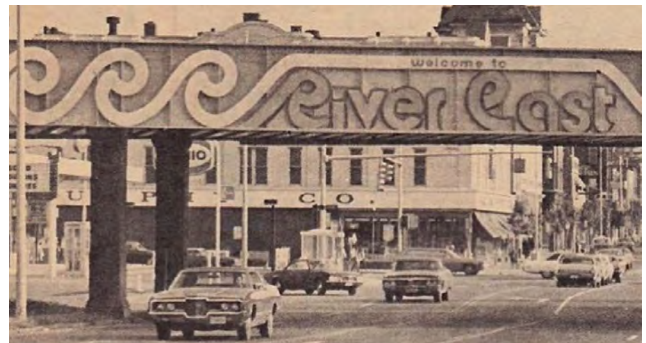
Image of previous rail line over Main Street, circa 1978
