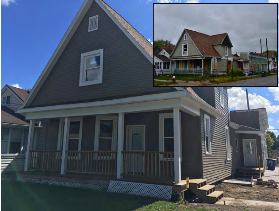
Home on the corner of Licking and Mott Avenue currently under renovation with NeighborWorks Toledo Region
