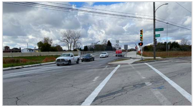
Dorr Street Overpass
