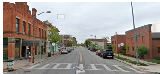
Existing Condition - Adams Street
