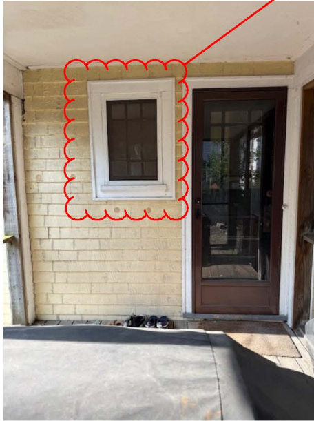
Exterior view from interior of the screen porch
