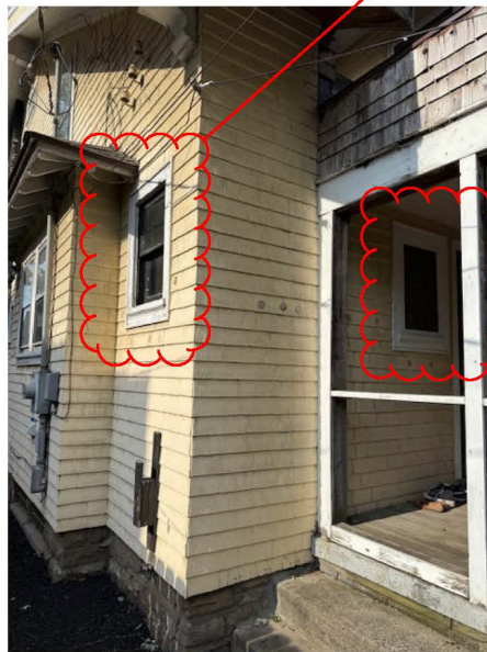
Exterior view of the southwest corner
