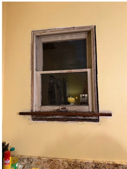
Interior view (southwest corner)
