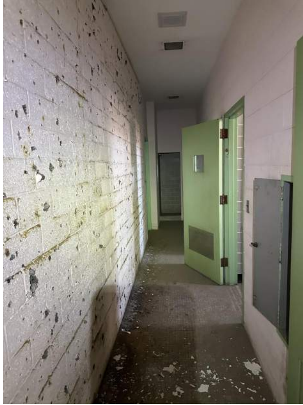
Architecture/Structural – Typ. Interior Block Moisture Blow-outs
