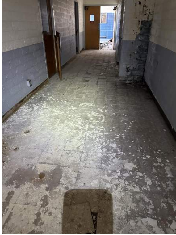
Architecture – Asbestos Floor Tile
