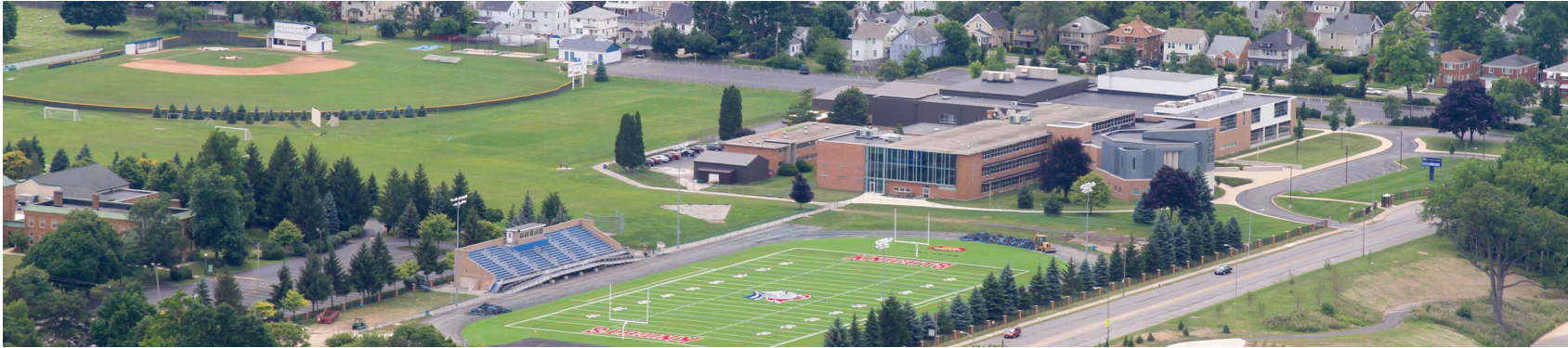
E1 EXISTING CAMPUS PHOTO SCALE: 1:2.51
